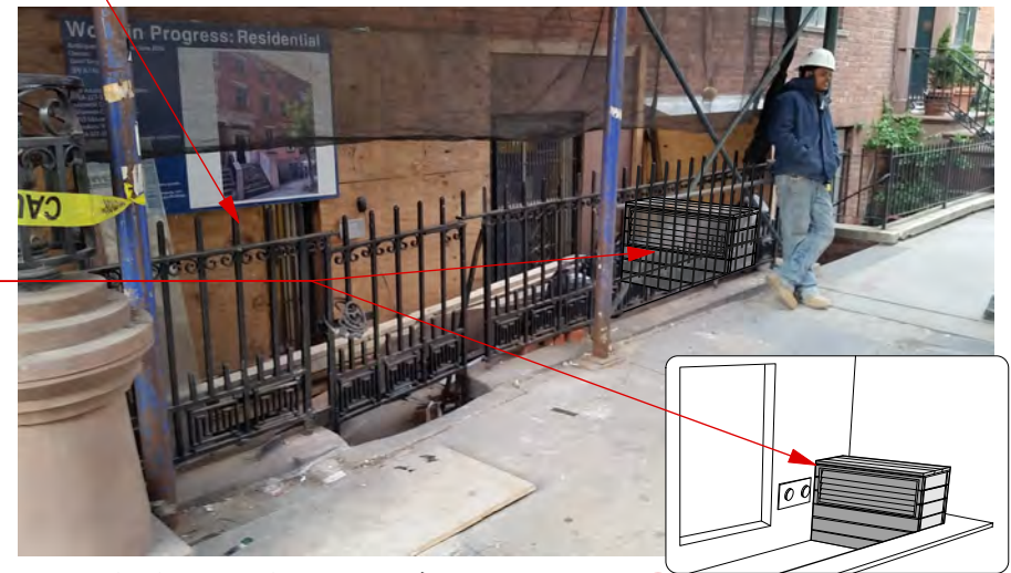
D. IPE-WOOD AIR-INTAKE ENCLOSURE, RAILING OMITTED FOR CLARITY
