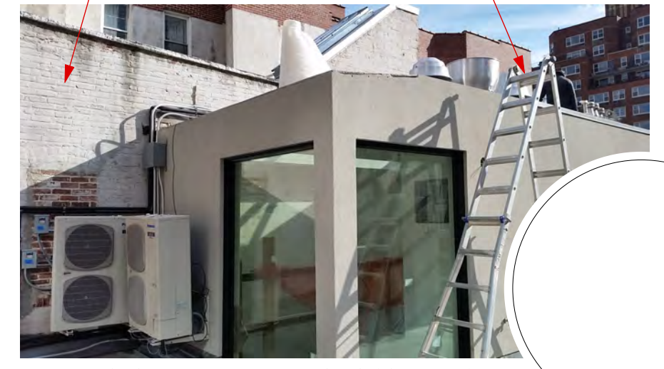
A. RELOCATED MECH. UNIT - (NOT VISIBLE IN PHOTO, OUT OF LINE OF SIGHT FROM STREET) FORMER LOCATION OF MECHANICAL UNIT
